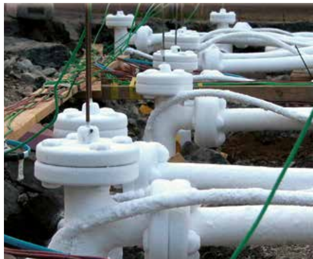
The soil freezing system in operation
