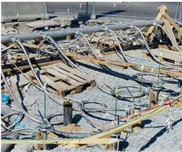
The soil freezing system under construction
